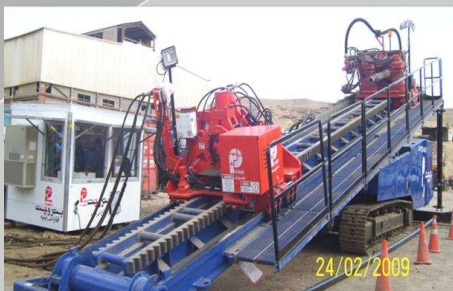
Horizontal Directional Drilling
